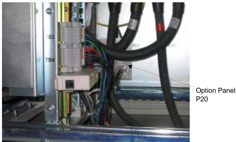
Figure 2-10 GT100E MS Interface Assembly Cable Connection
